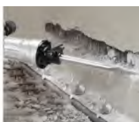
The walls were torn down
