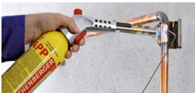
Brazing in gas installation
