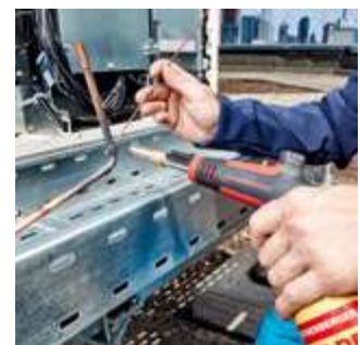
Brazing in refrigeration / air-conditioning technology
